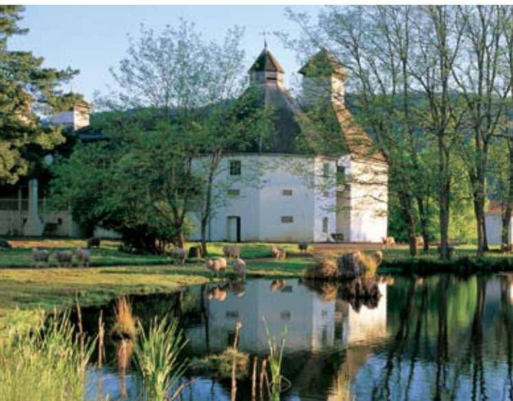
Cast House, Derwent Valley
